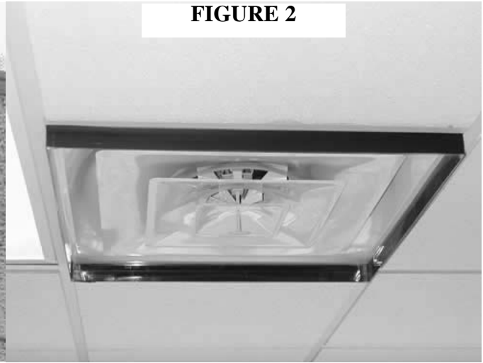
CLEAN CEILING TILES WITH AIRTECH CTP (CEILING TILE PROTECTOR SHOWN ABOVE IS BLACK FOR ILLUSTRATION PURPOSES ONLY)
